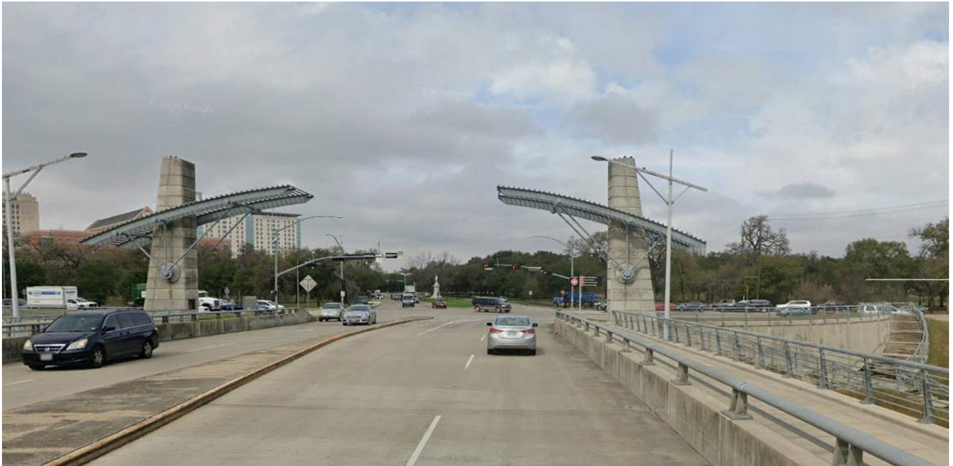
Photos at Other Area Brays Bayou Bridges – Cambridge Street Richard E. Wainerdi Bridge
