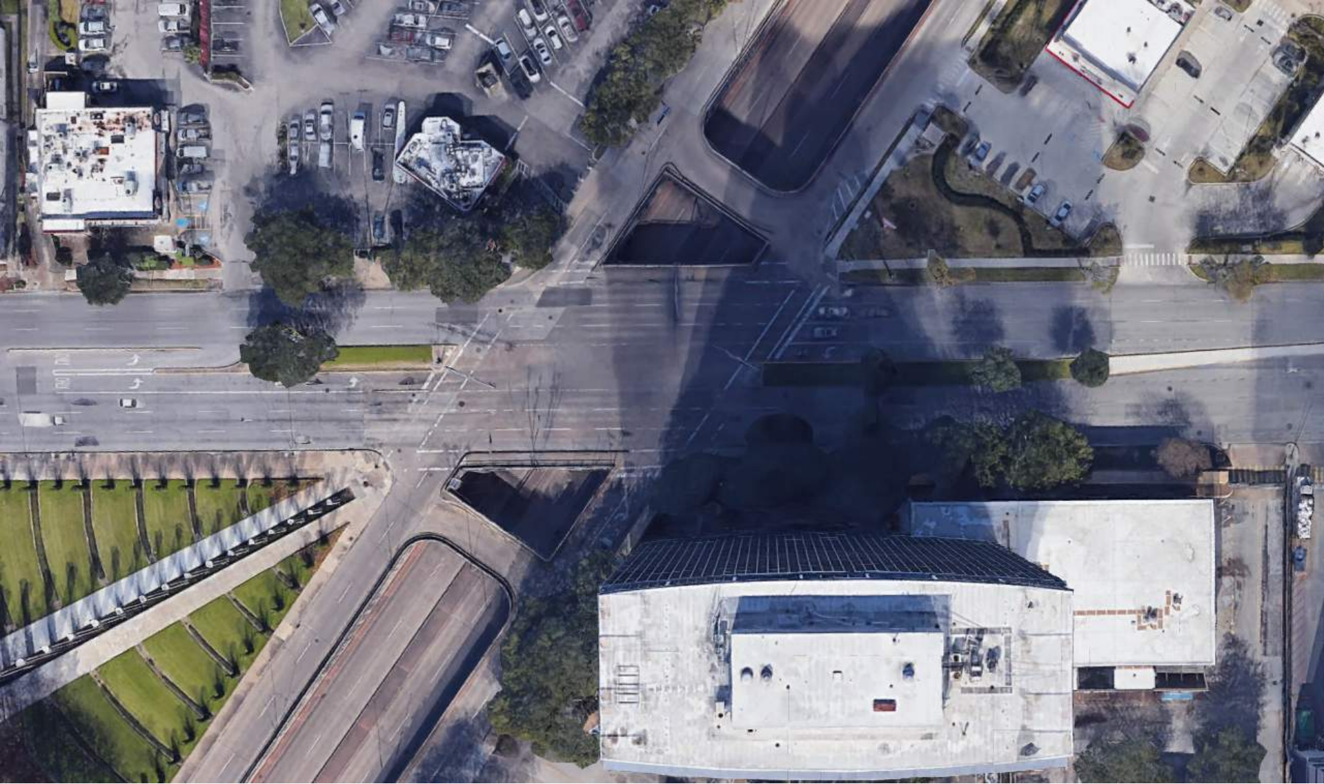
Holcombe Boulevard at Main Street Area Aerial Detail
