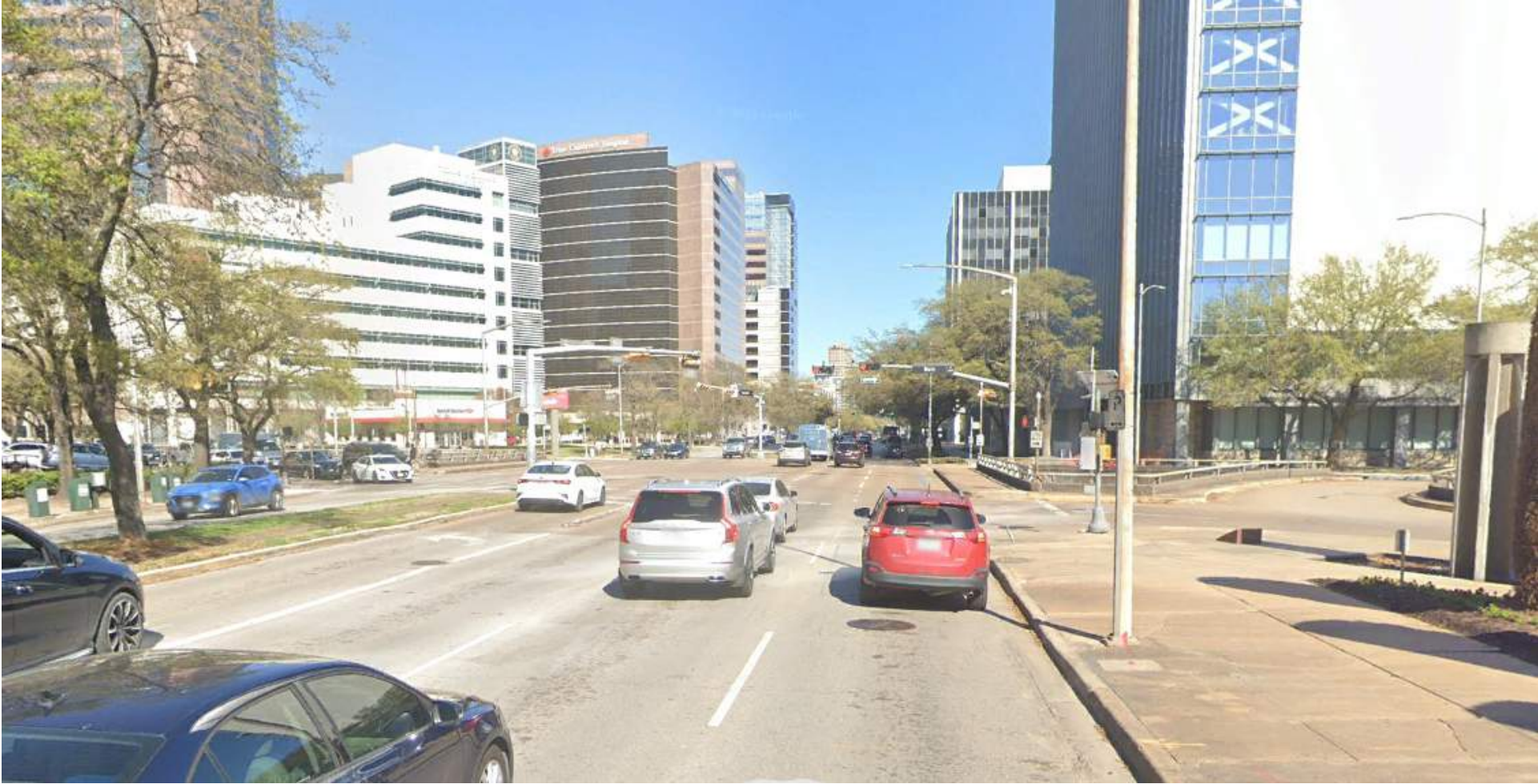
Holcombe Boulevard Looking East at Main Street
