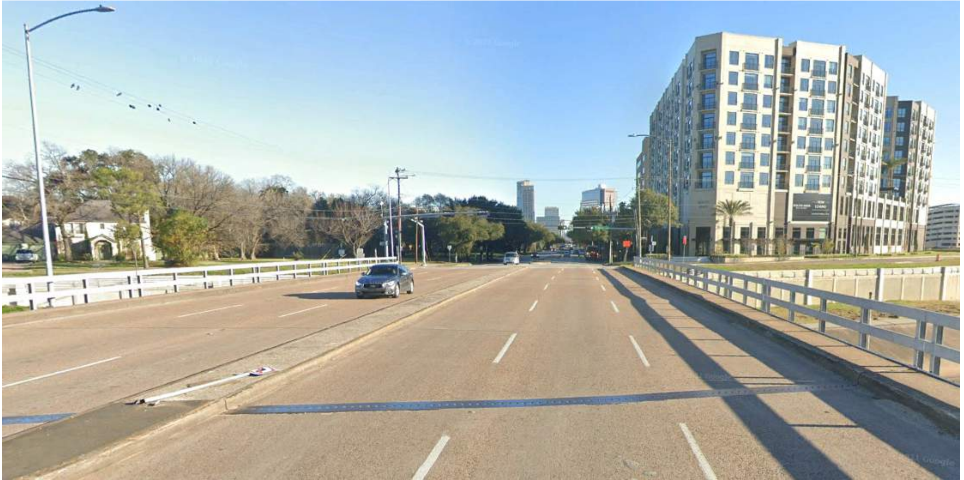
Main Street Looking North on Brays Bayou Bridge
