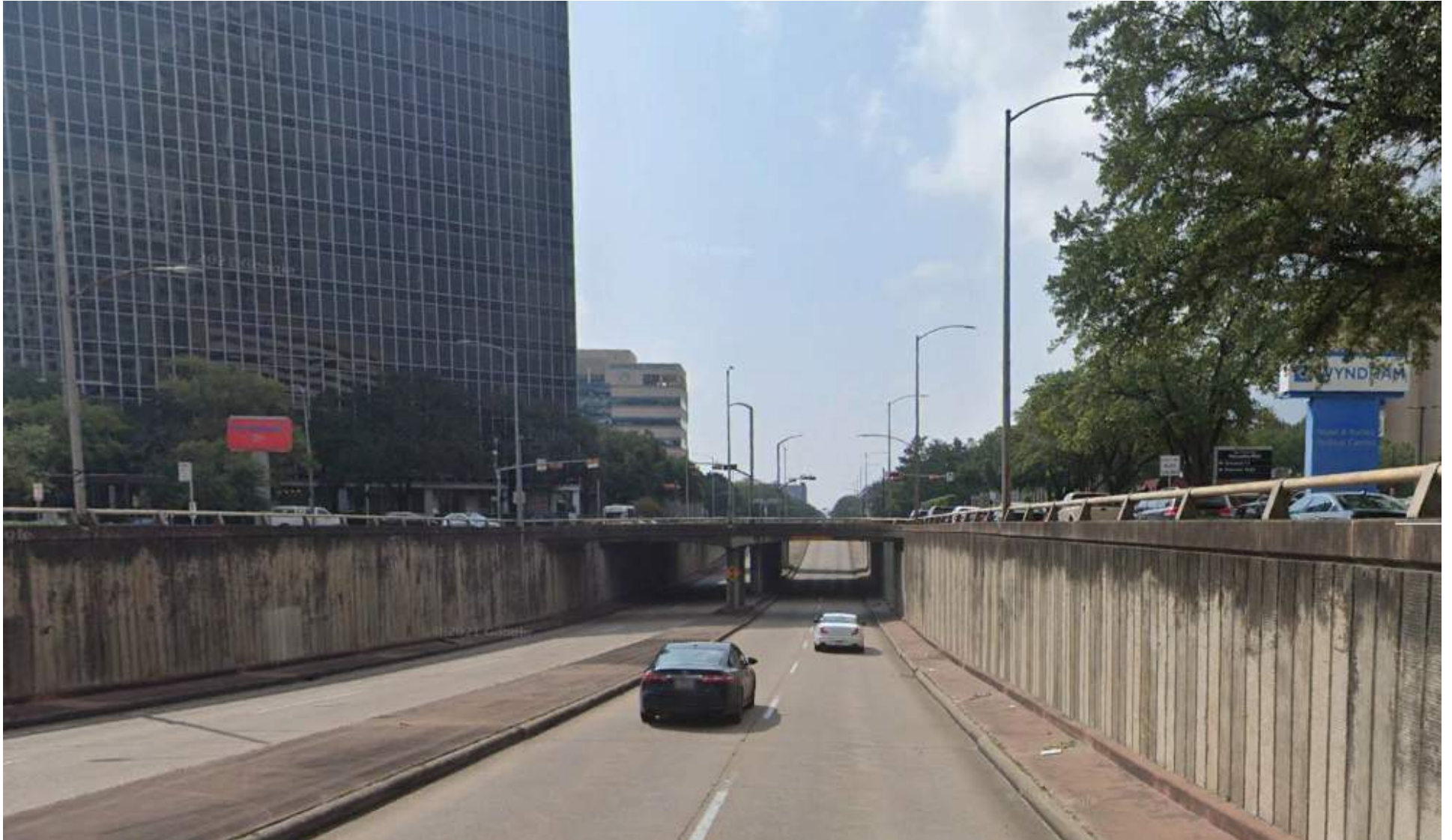
Main Street Underpass Looking South at Holcombe Boulevard
