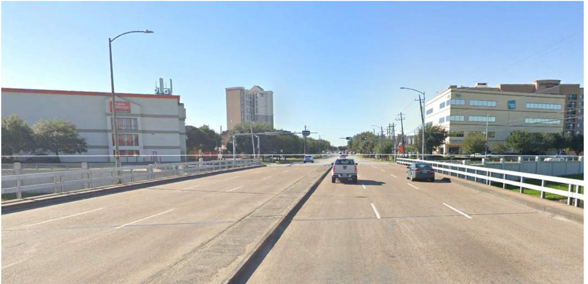
Main Street Looking South on Brays Bayou Bridge
