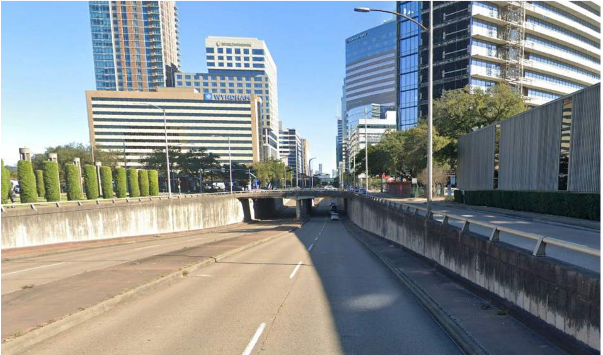
Main Street Underpass Looking North at Holcombe Boulevard
